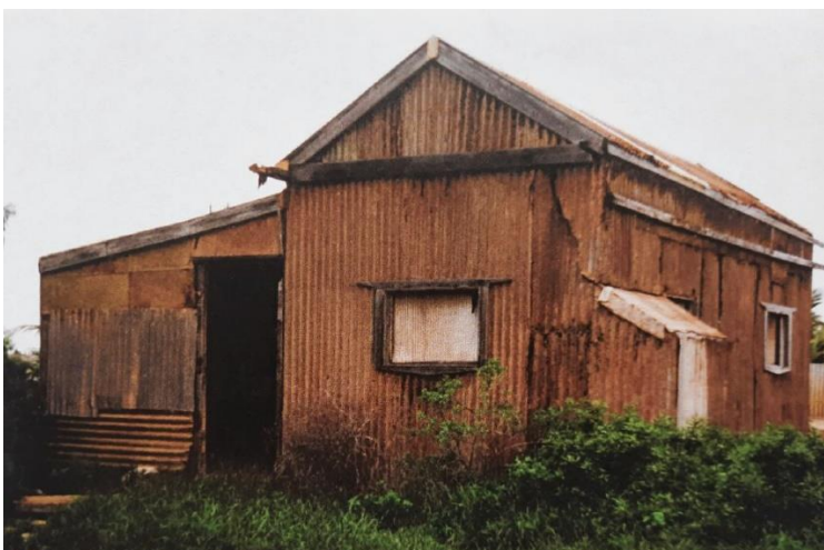
Figure 3 - "French's Shack" constructed 1933
