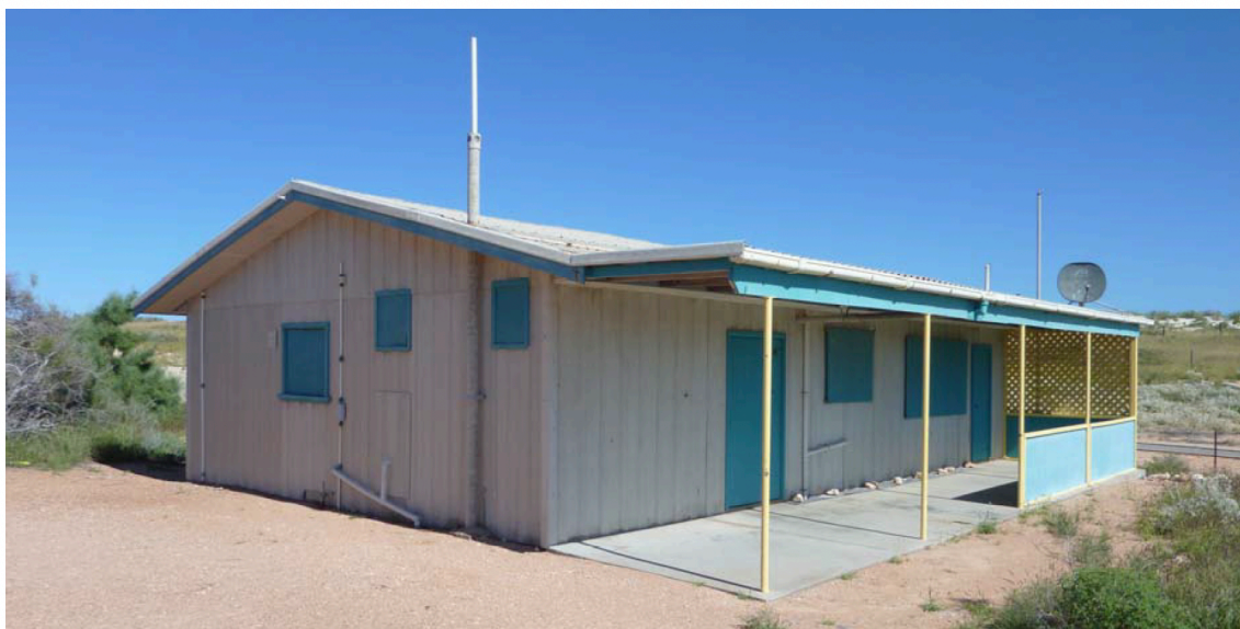
Figure 8. Building on Lot 54 called French's Shack. (Shire of Carnarvon MHI 2015, p. 229)
