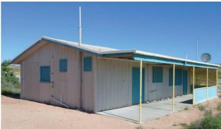
Figure 1 - Existing Asbestos Building
